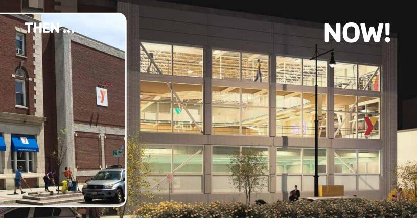
**Structural and façade improvements** will bring vibrancy to North Street. Drafty and bricked up windows will be replaced with energy efficient glass to let natural daylight in. Failing mortar joints will be repointed at the façades on North and Melville Streets. LED lighting, and an energy-efficient heating and cooling system will conserve energy.
